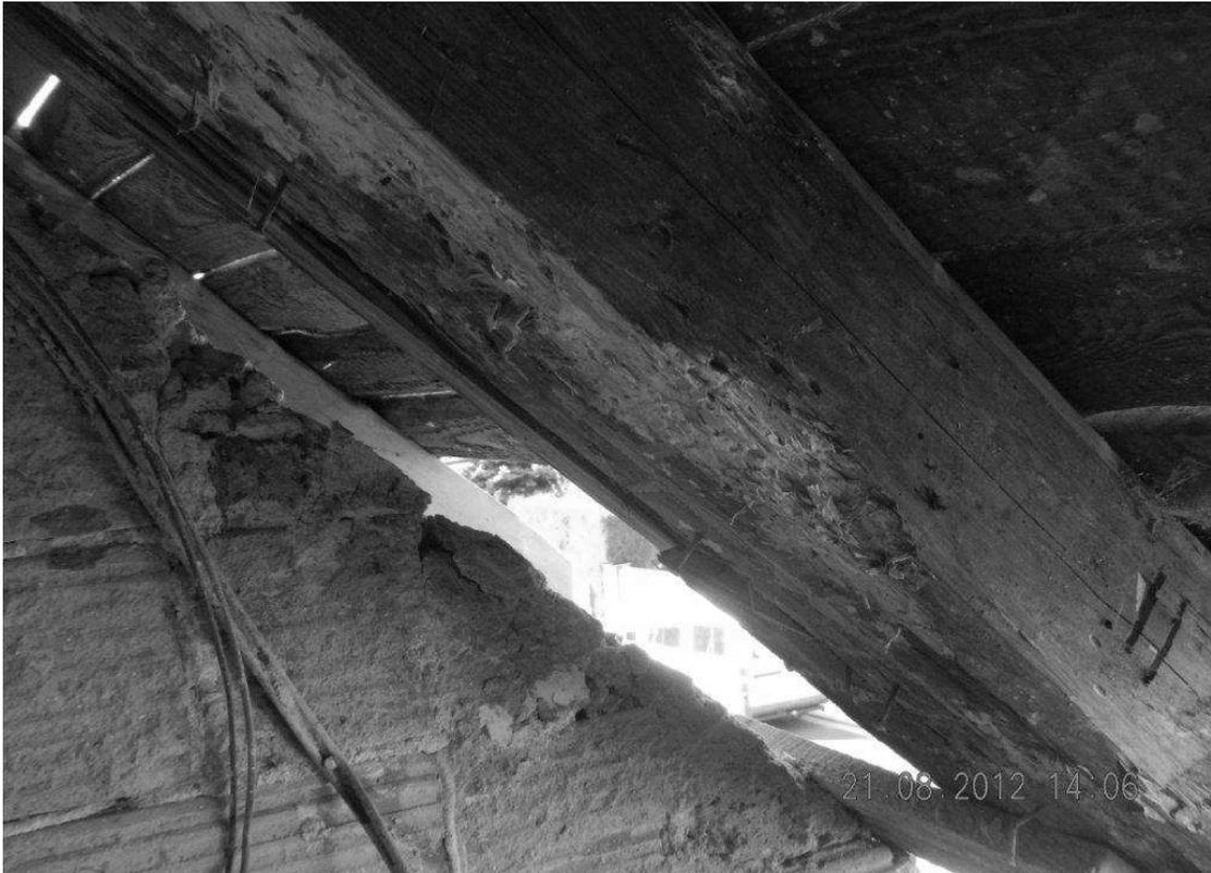
Figura 3 - Photograph of an example of wood-destroying insect action
