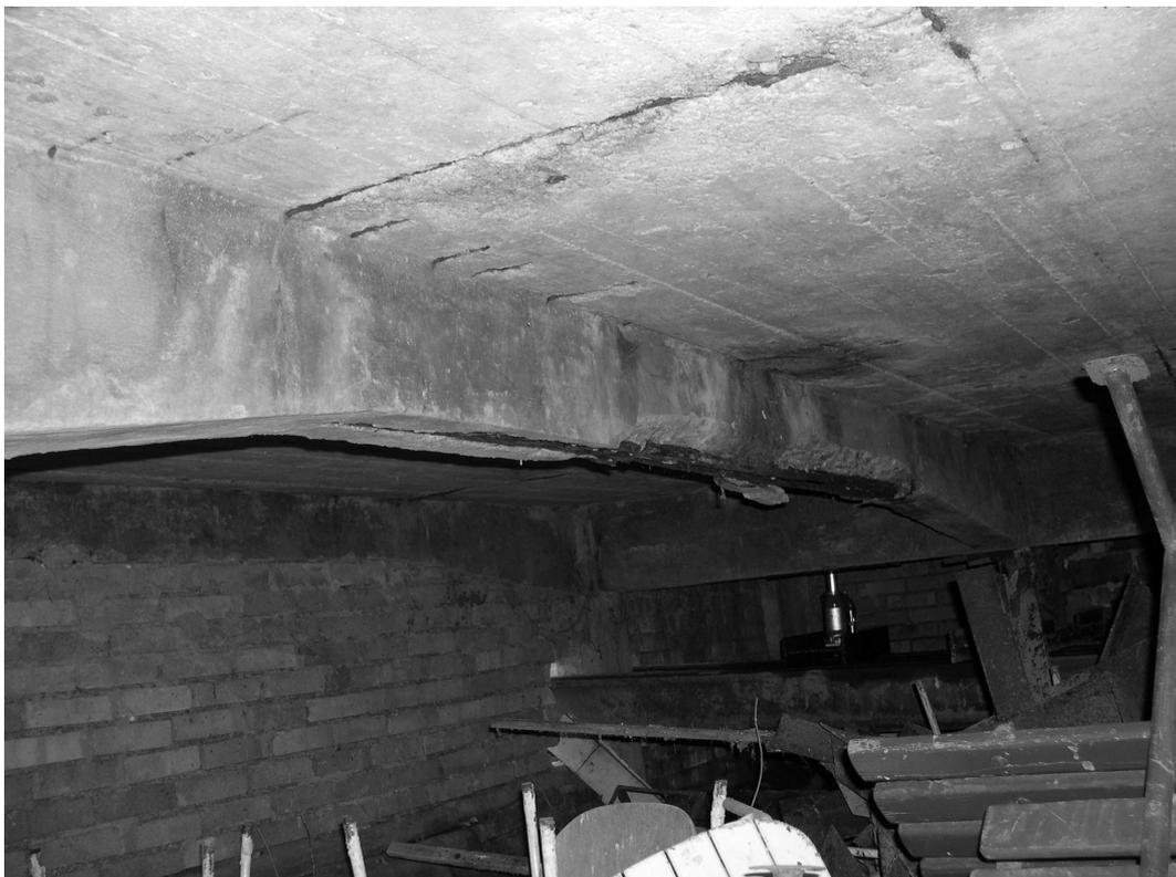
Figure 5 - damage to the reinforced concrete beam and slab
