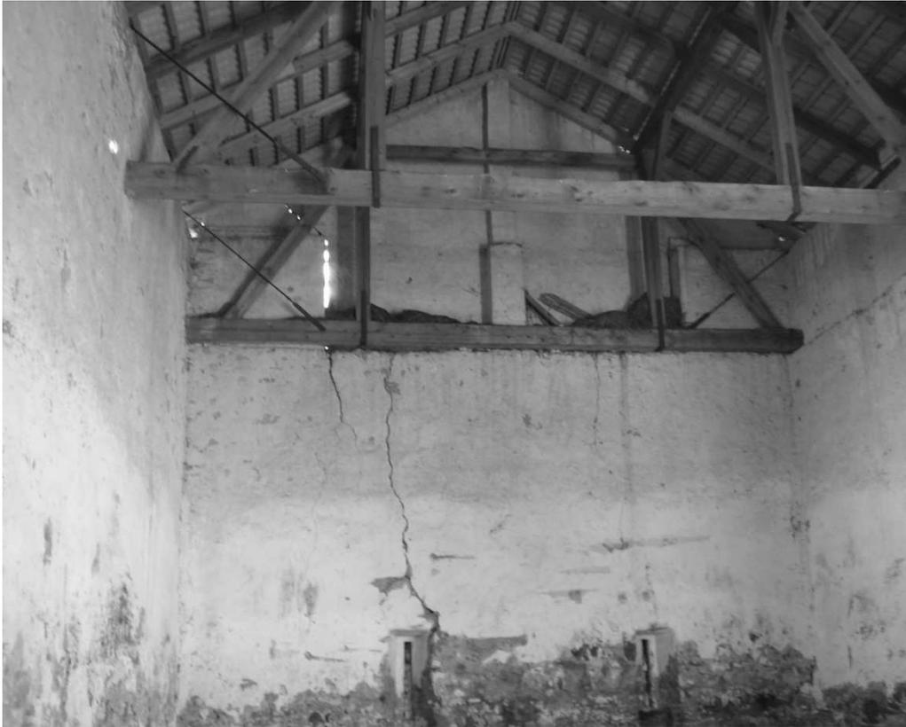
Figura 2 - Photograph of failures in the masonry
